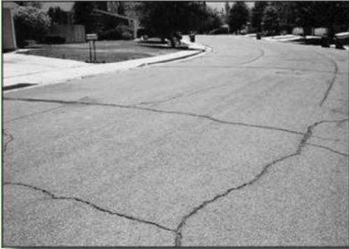
For medium-volume roads, this may mean a minimum HMA thickness of about 11 inches, and for heavier trafficked roads, it could mean structures of 15 inches to 16 inches at the thickest. Of course, the thickness in a given situation depends upon the traffic, soil, foundation and climate.
